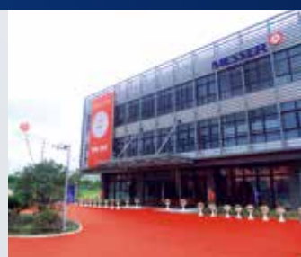
Completion of the second building phase in China
