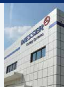
Foundation of Messer Cutting & Welding, China
